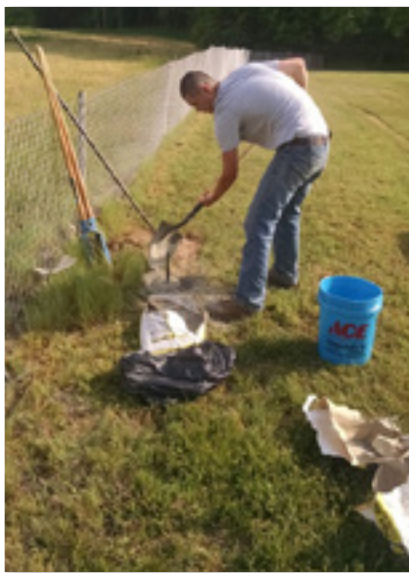
Installing the box.
