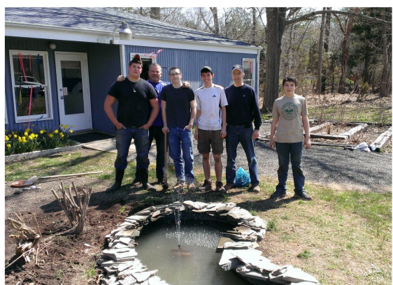
Scout members installing the fountain.
