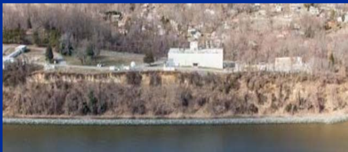
Cliff-side before project started.
